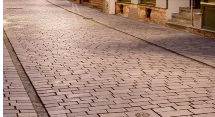
In ground lighting
